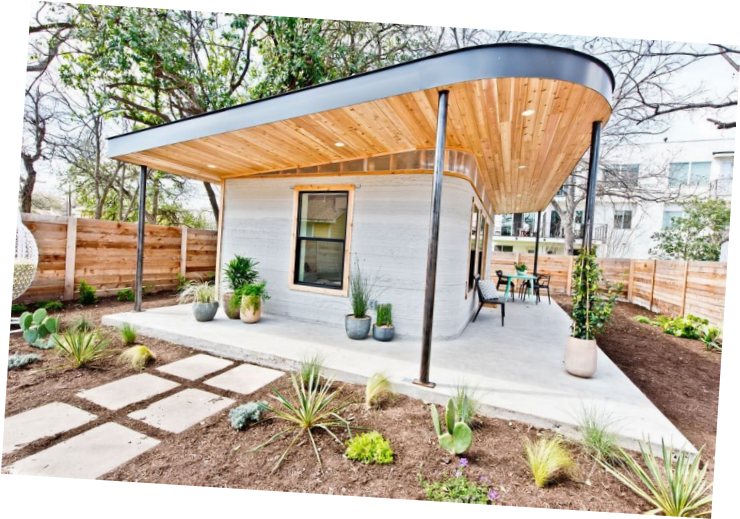
3 D Printed House Austin, TX 48 hours/$4,000
